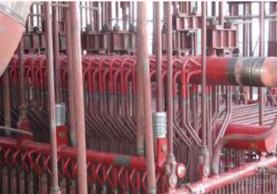
Power station boiler high temperature superheater
