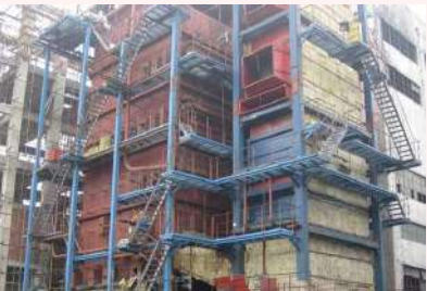
Power station boiler under construction
